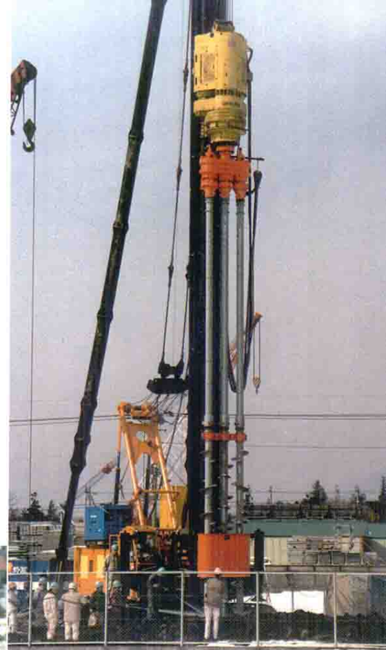
Upper left : TMW Drill head Upper right : State of driving operation (drive unit and drill stem) Middle left : Guide trench Center : Cement milk being ejected from the bits of both ends. Lower right : Exposed soil mix wall for visual inspection Lower left : Dug out soil mix wall body
