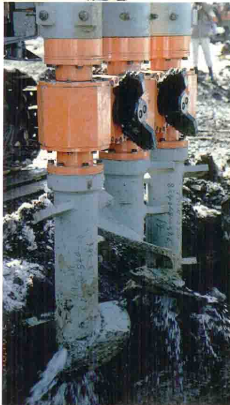
Upper left : TMW Drill head Upper right : State of driving operation (drive unit and drill stem) Middle left : Guide trench Center : Cement milk being ejected from the bits of both ends. Lower right : Exposed soil mix wall for visual inspection Lower left : Dug out soil mix wall body
