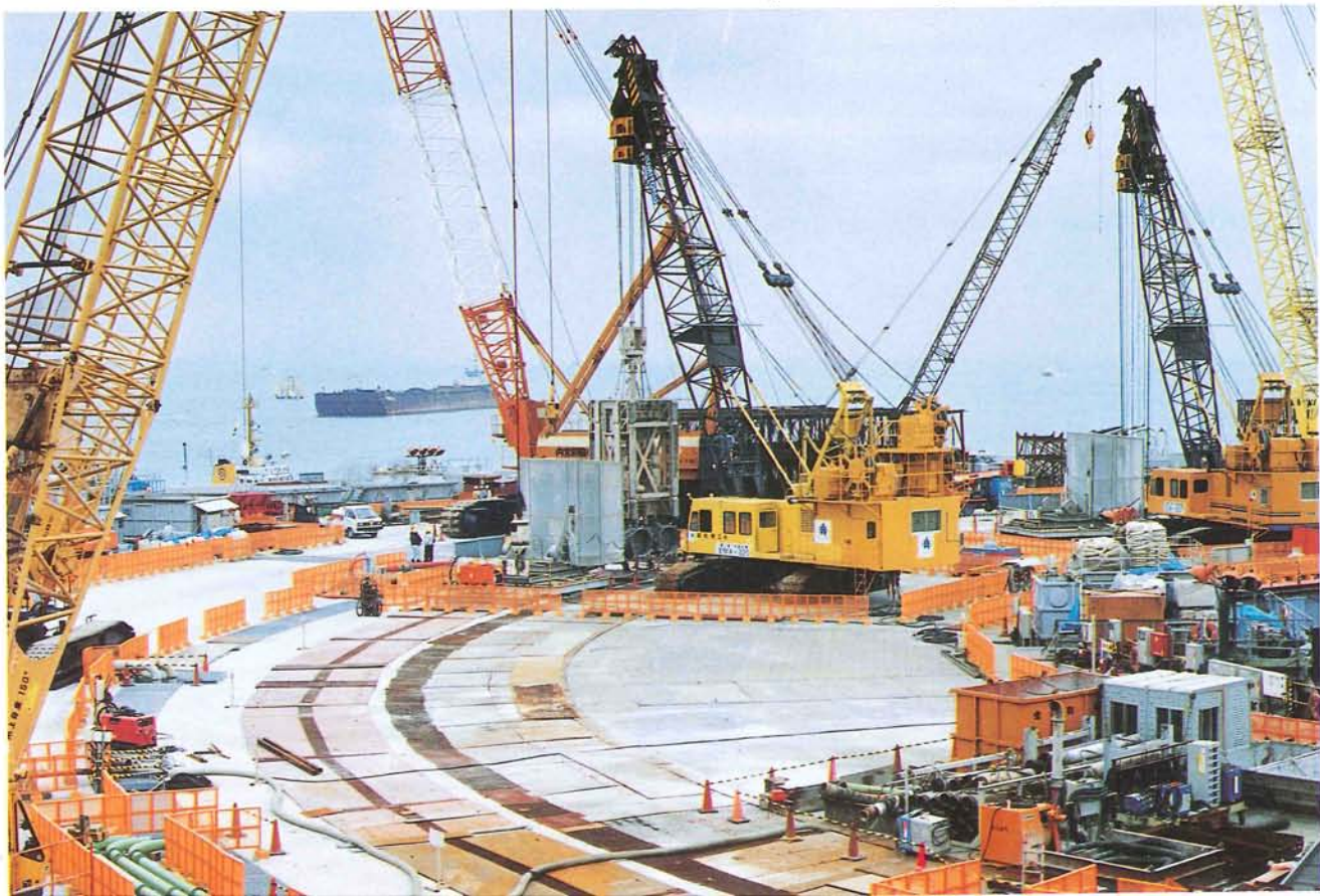
Two sets of EMX-320 drills are in operation in sight along circular guide walls.
