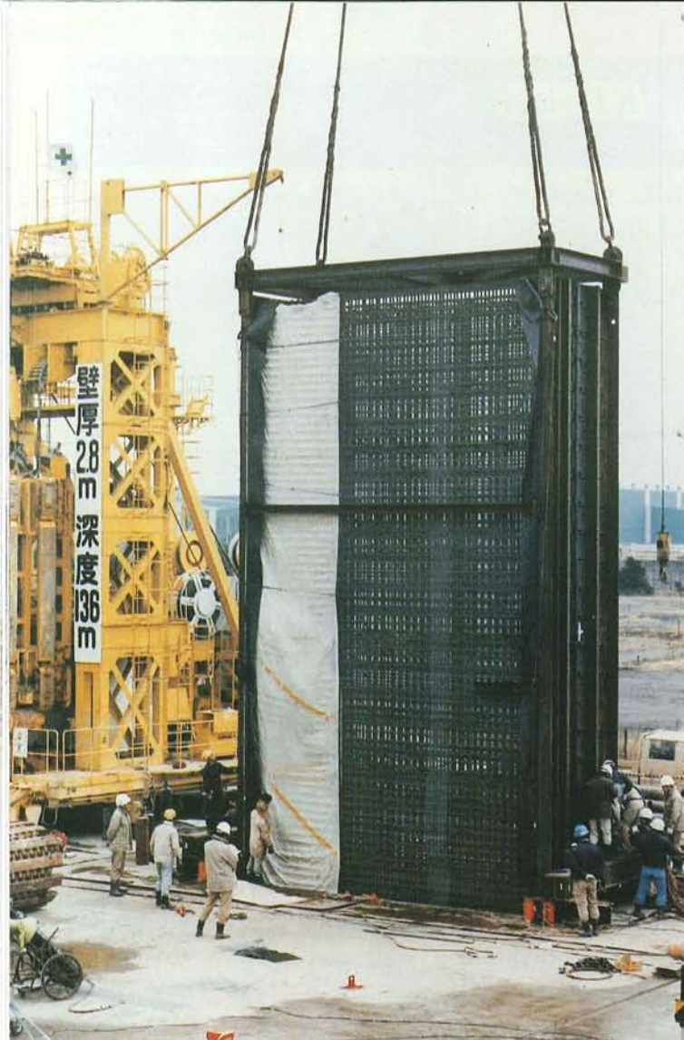
Real size test operation for 2.8 m wide and 136 m deep diaphragm wall construction conducted on the land prior to main construction.
