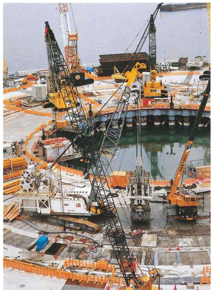
General view of ring shaped island with 3 units of EMX-320 drills in sight.
