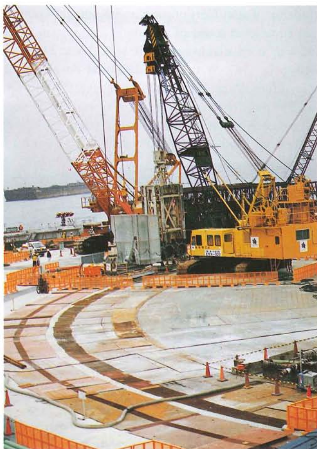
EMX-320 Drill in operation along circular diaphragm wall alignment.
