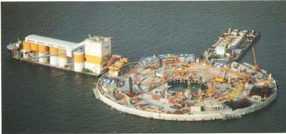
Aerial view of Kawasaki man-made island with anchored barges for stabilizing solution and concrete plant.
