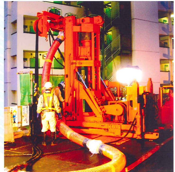
Photo of job site operating Down-the-Hole Bit along with "TBH" base machine
