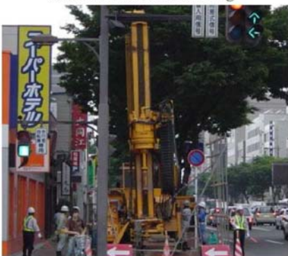
Geothermal hole drilling
