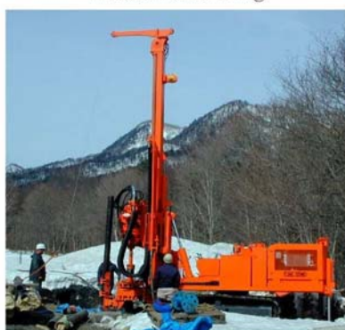
Water well drilling
